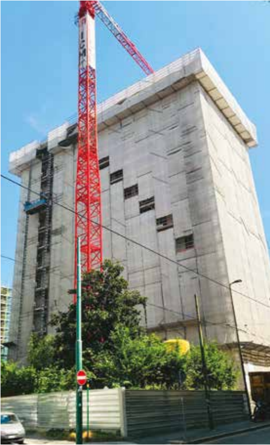
General redevelopment of the hotel complex called "The Big" on behalf of Unipol Sai Spa in Milan
