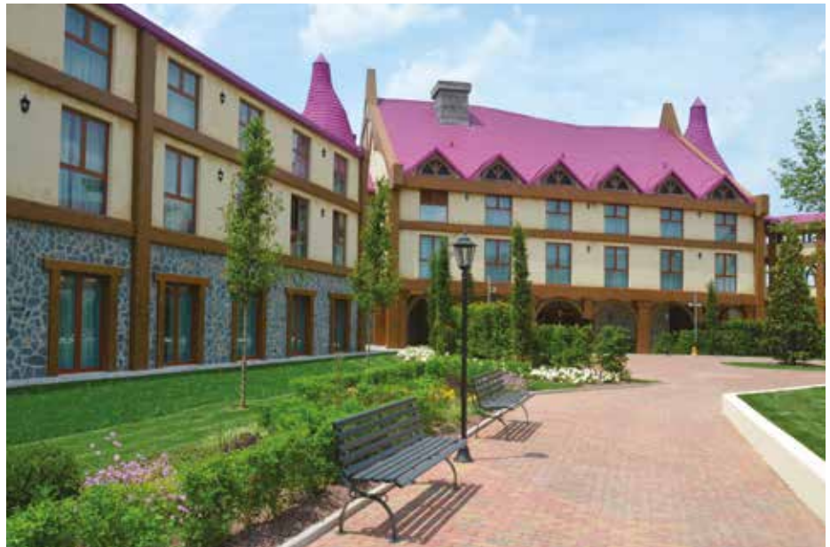
Construction of Gardaland Magic Hotel, new themed tourist complex in Castelnuovo del Garda (Verona)
