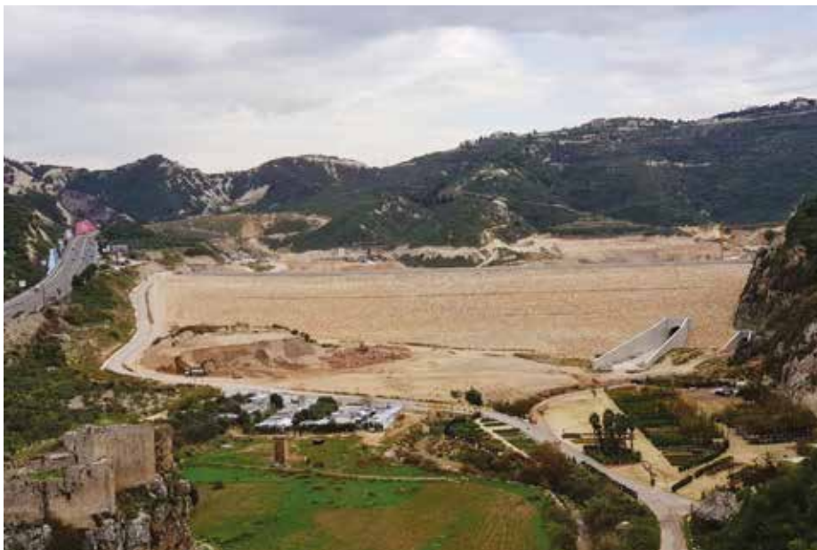
Construction of the Mseilha dam in the Republic of Lebanon on behalf of the Ministry of Energy and Water
