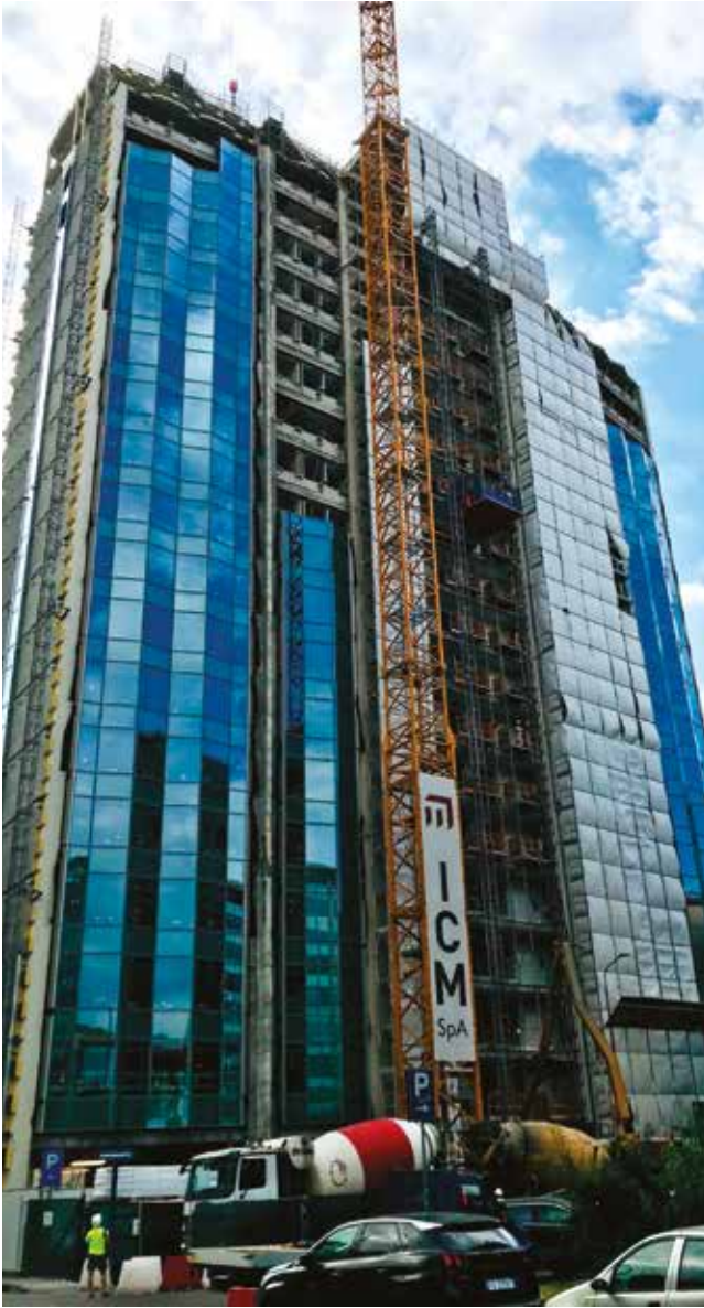
Construction, on behalf of Coima, of "Corso Como Place", an office and commercial complex in the Porta Nuova area of Milan
