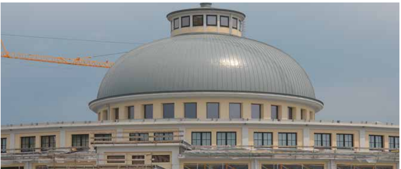
Restoration and redevelopment of the former "La Rotonda" ice production plant in Verona
