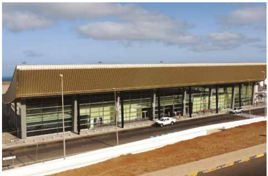
Expansion of the Praia Airport, in Cape Verde, as requested by the Ministry of Infrastructure
