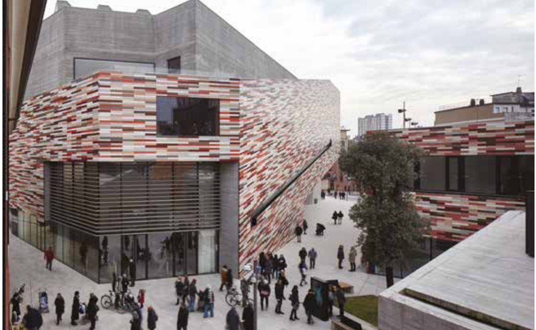
Construction of the New Cultural Complex and the Museum of the Twentieth Century (M9) near Venice-Mestre
