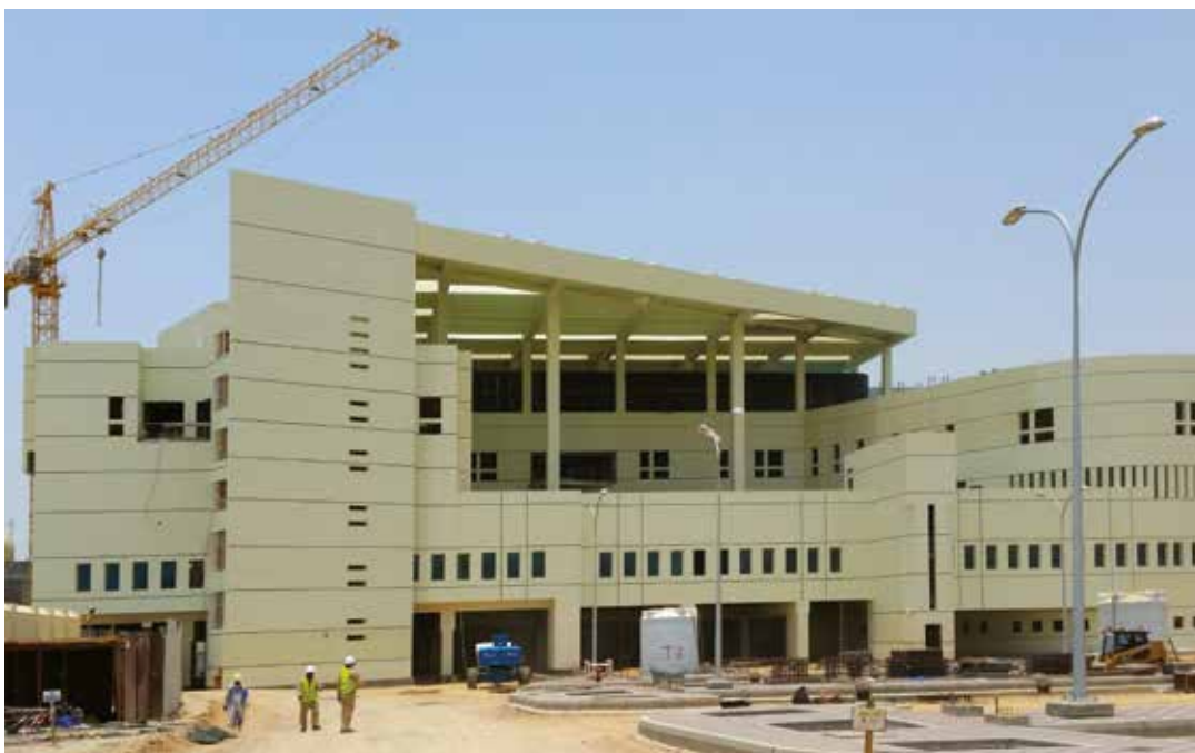
Construction of the Al Khoudh Military Hospital in the Sultanate of Oman on behalf of the Ministry of Defense
