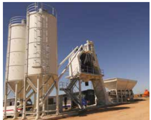
Design and construction of the infrastructure for the development of the new Smart City of Konza, in Kenya: the future Silicon Savannah
