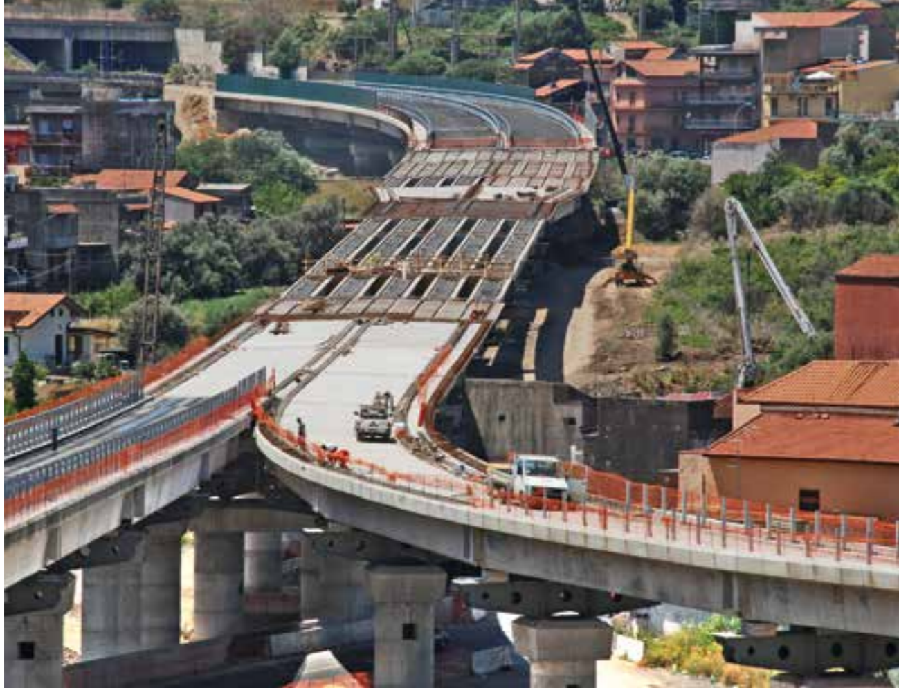
Dual carriageway, Catania
