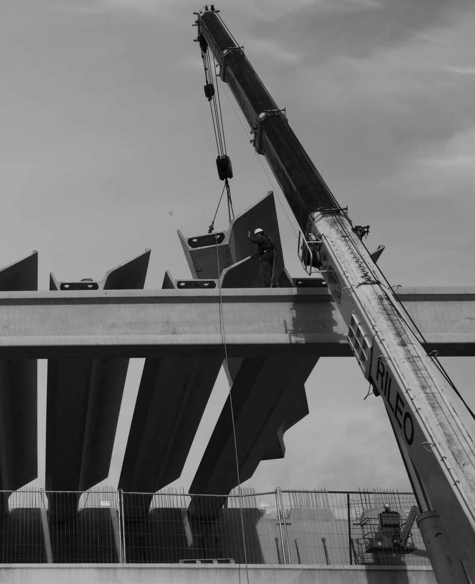
Assembly of prefabricated installations in the building site Progress-OVEG in Prato allo Stelvio (BZ)
